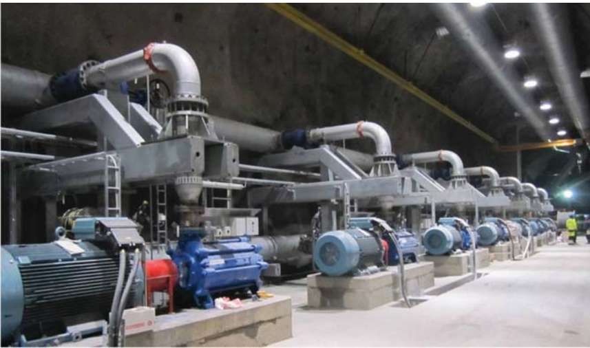
Every day 76,000 tons of ore are brought to the surface in the Kiruna mine alone, part of the LKAB company, which is roughly equivalent to the volume of a 12-story building.
