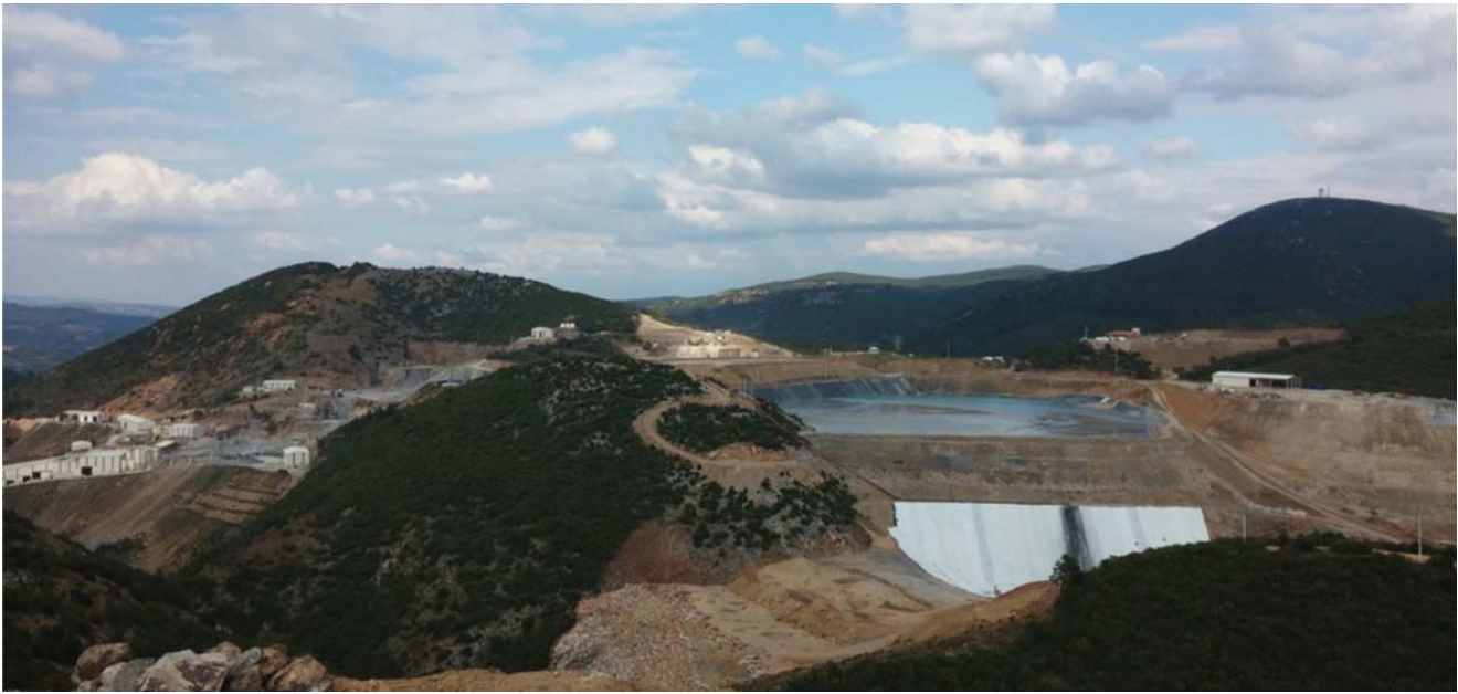
Eczacıbaşı Esan Lead & Zinc Facility is operating a very old mine (500 BC) around Marmara region in Turkey. Raw ore extracted from an underground lead and zinc mine is processed at crushing, milling, and flotation facilities.
